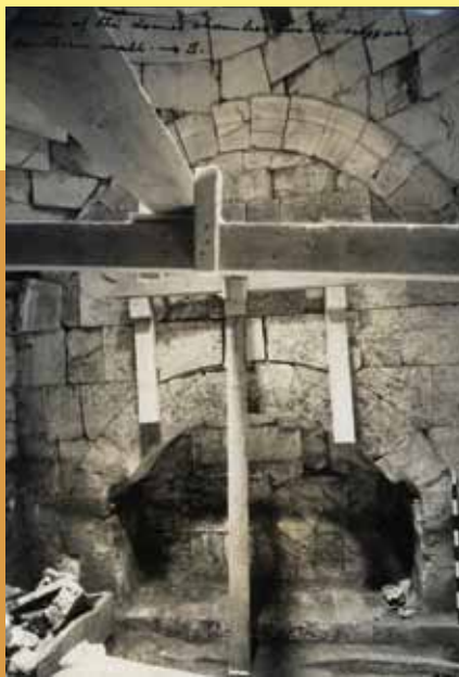
Interior of the domed tomb before demolition
