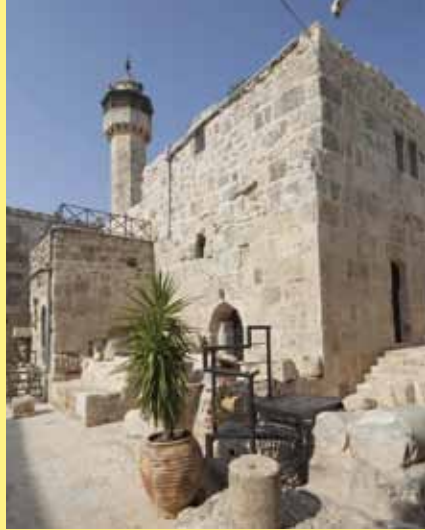
The renovated area
