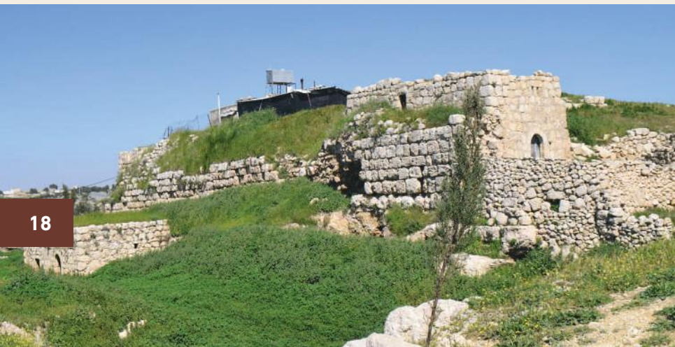
Citadel's western wall before conservation works.
