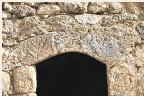
Segmental arch with ancient stones in the front door of a simple-type house.
