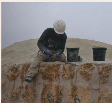
During conservation works outside the coffee shop
