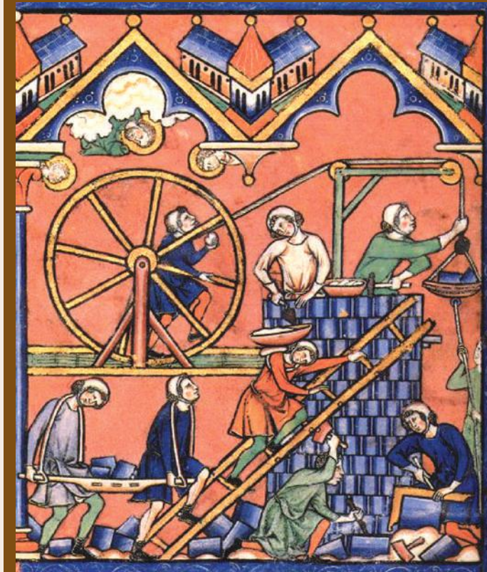
The use of a treadwheel crane and other devices in the building of a tower in a 13 th -century drawing
