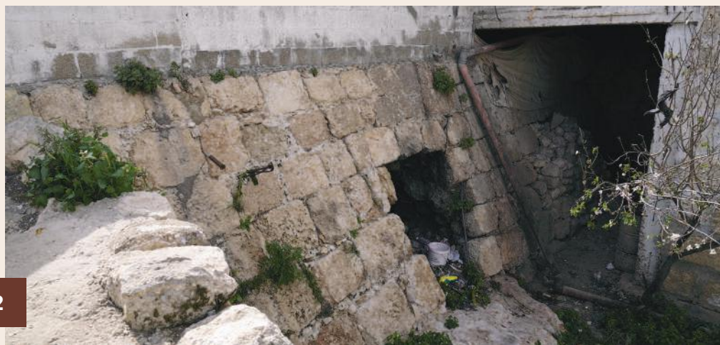
Glacis in the northern part of the tower inside Al-Burj Citadel
