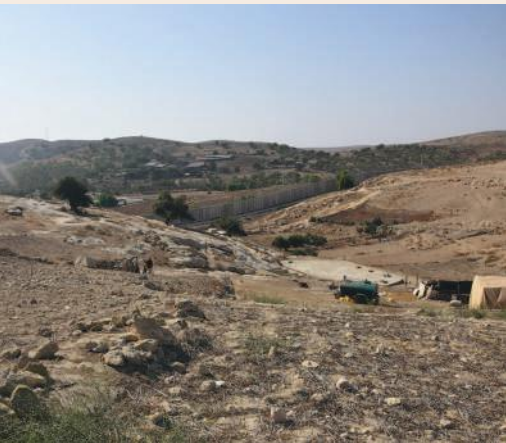
The area of Abu Touq Pool covered with a concrete slab
