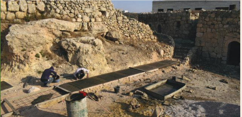
During the construction of the ramp
