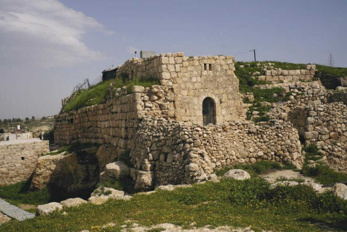
General view of the Citadel with the west wall after restoration and the moat.
