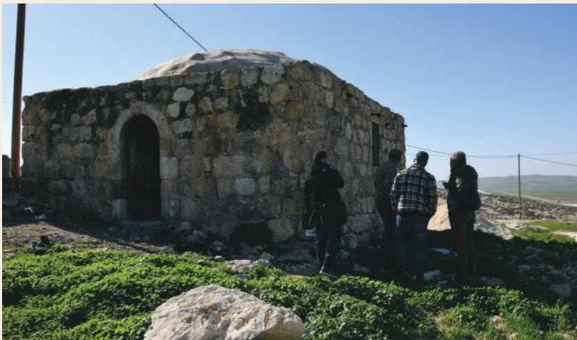
The coffee shop before conservation works
