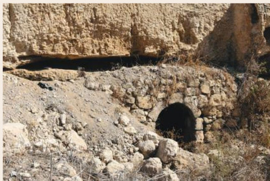
Cave dwelling inside the northern part of the moat of Al-Burj Citadel.
