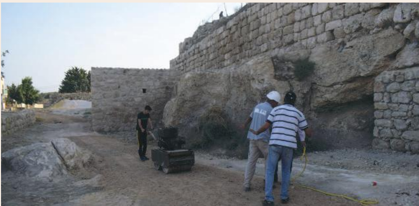
During the construction of the ramp
