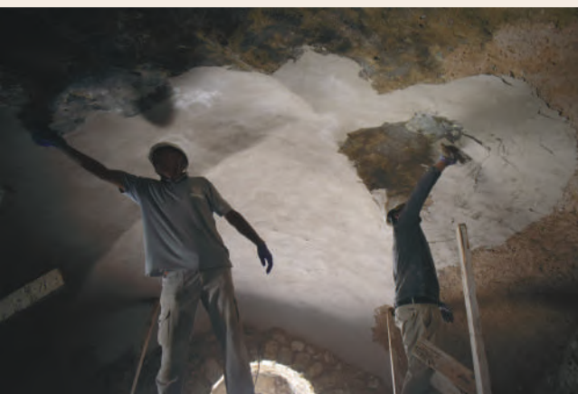
During conservation works inside the coffee shop
