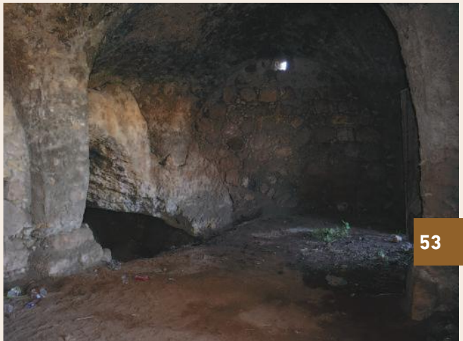
Inside the Storytelling house before conservation works
