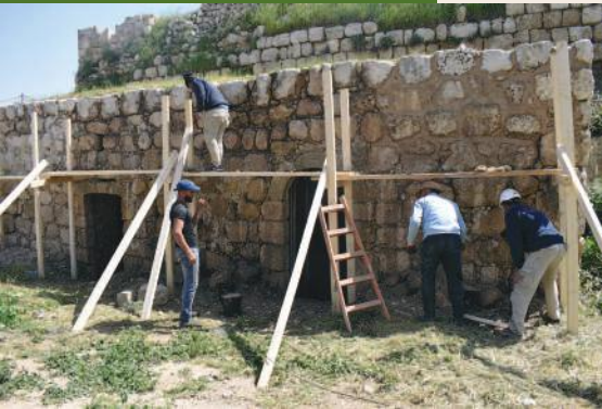
During conservation of the façade of the Storytelling house
