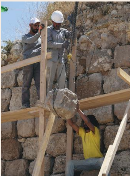
During the reconstruction of the Citadel.
