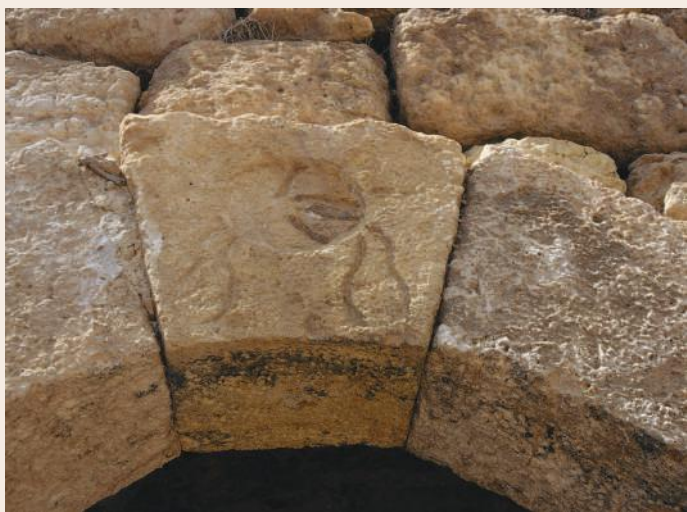
Detail of an ancient stone, reused in the arch of the door and decorated with birds.
