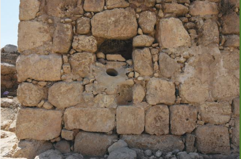
A zeer incorporated into the courtyard wall to keep the drinking water cool
