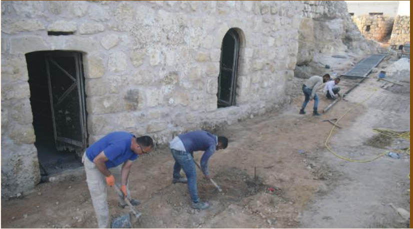
During the construction of the ramp
