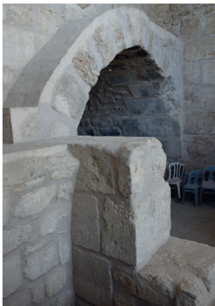
Above: Arched substructure that supported the south aisle of the fourth church.
