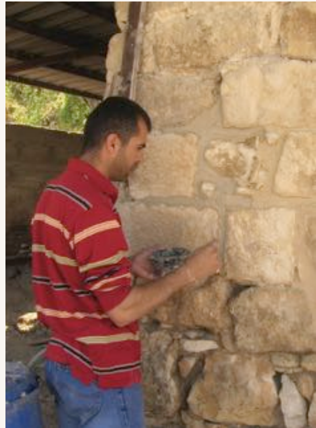
Setting of joints among stones
