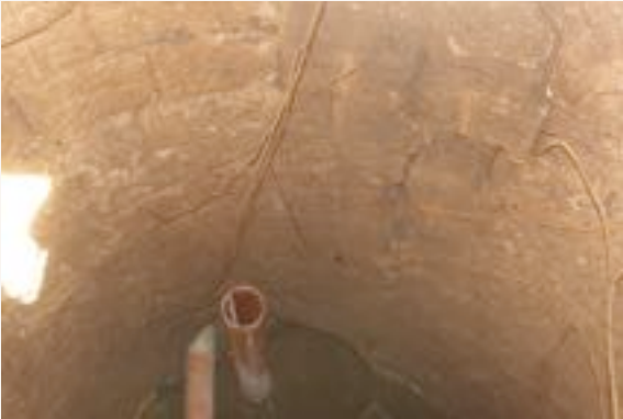
The interior of the well
