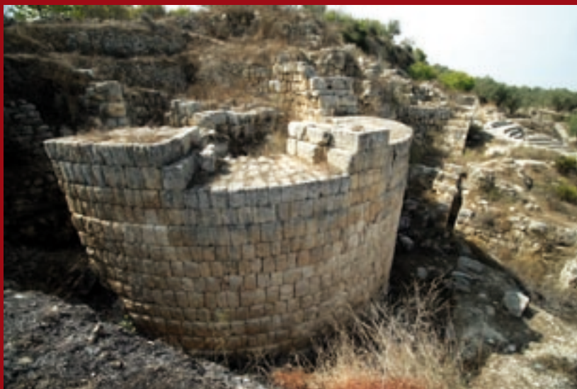
In the Hellenistic tower, all the stones are set on the head to strengthen the defense
