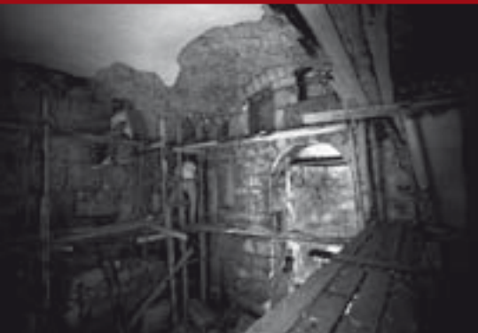
Workers in the new chapel
