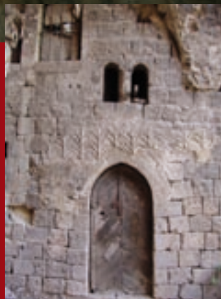
Detail from the traditional lime work on the Ottoman palace (XVIII century), Qasr al Kaid
