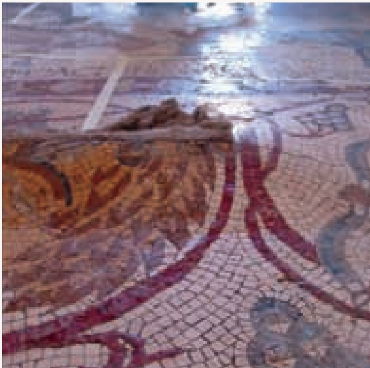
Swelling in the central nave
