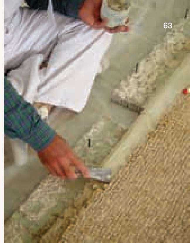
Setting of compatible mortar
