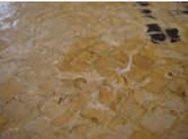
White cement over the mosaic surface
