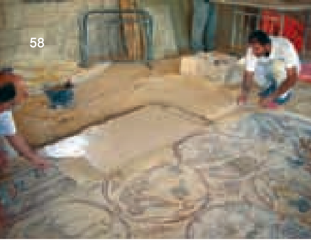
Preparing the foundation to relaid the mosaic
