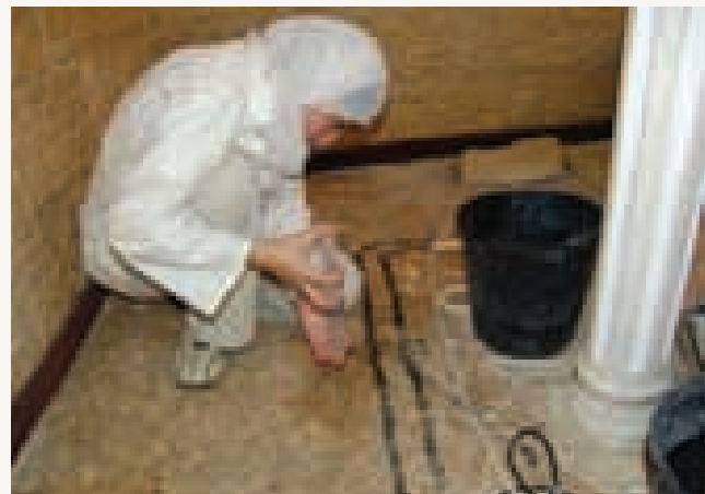
Consolidation by injection
