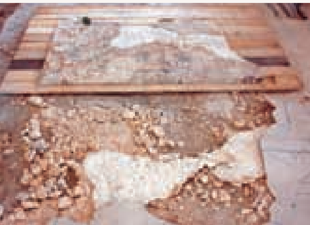
Just after lifting
