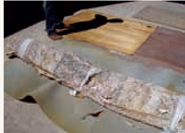
The condition of the mosaic before the intervention
