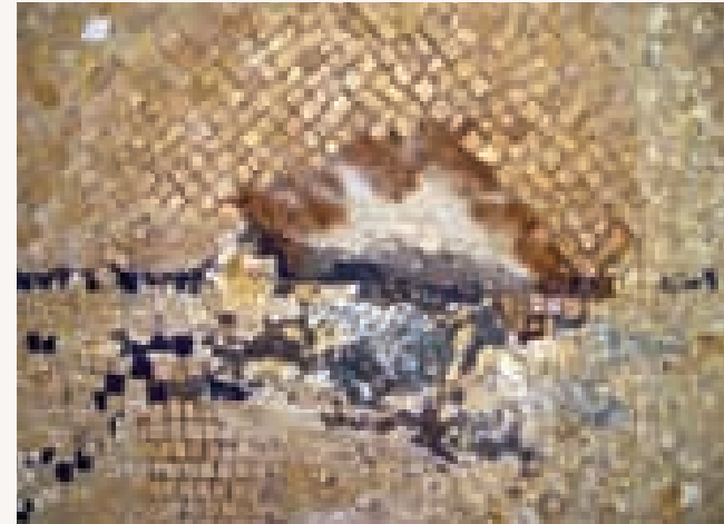
Black cement intervention
