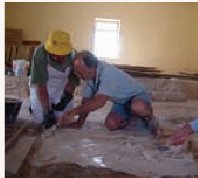
Preparing the foundation to relaid the mosaic
