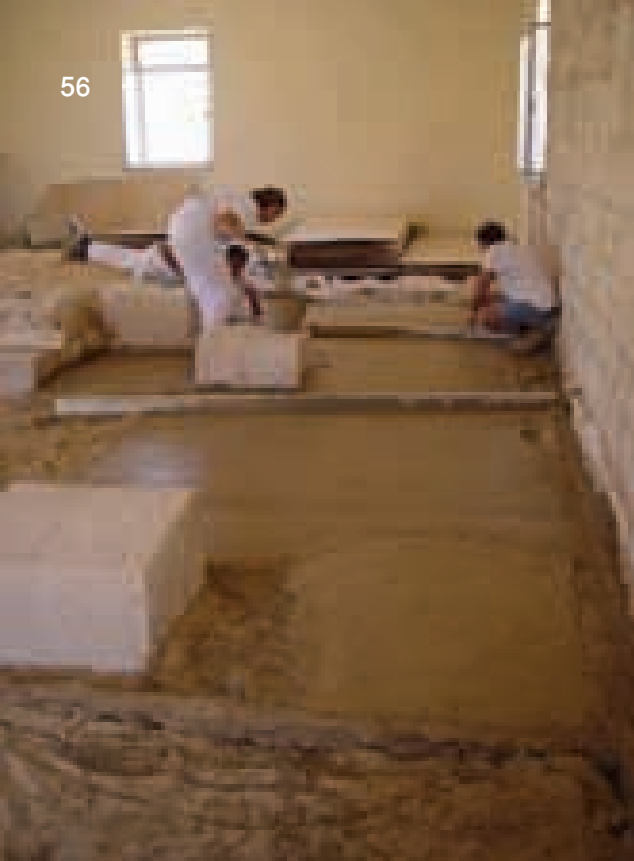
Preparing the foundation to relaid the mosaic
