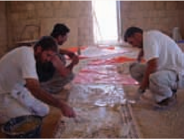
Preparing the bedding of the mosaic
