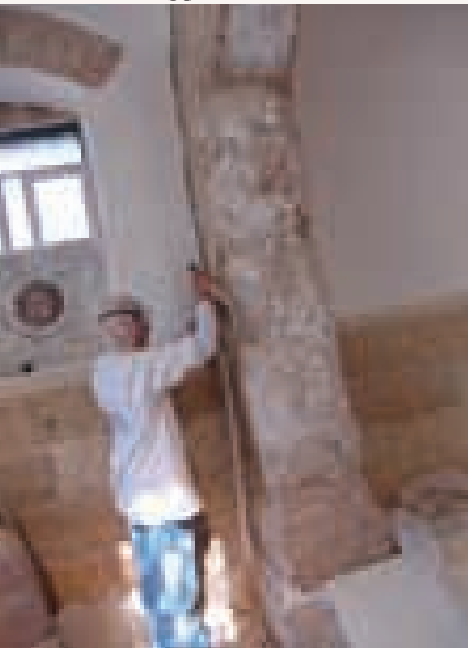
Removing plaster
