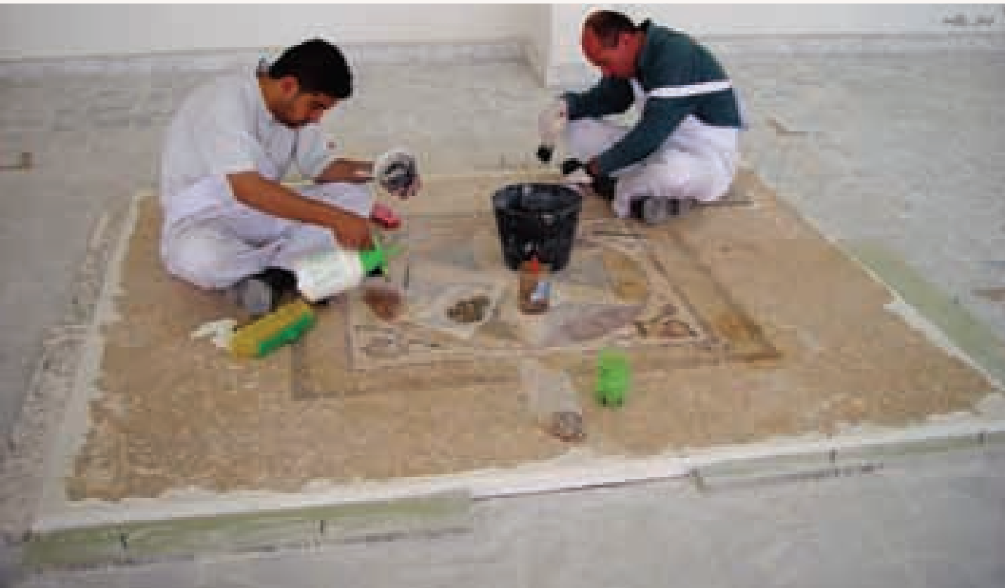
Cleaning after assembling the mosaic
