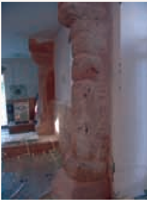
Internal view after plaster removal
