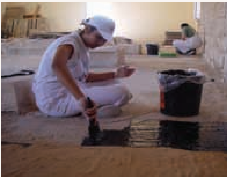
Preparing the foundation to relaid the mosaic
