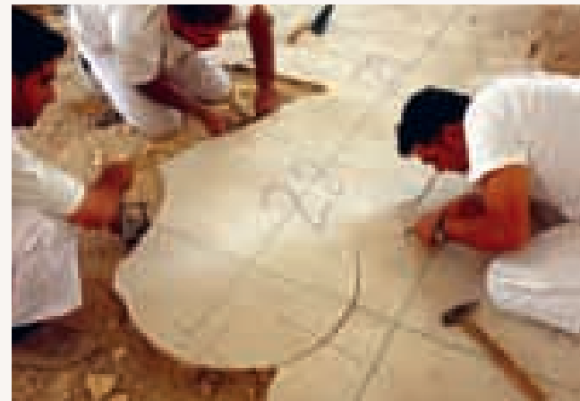
Preparing the mosaic lifting
